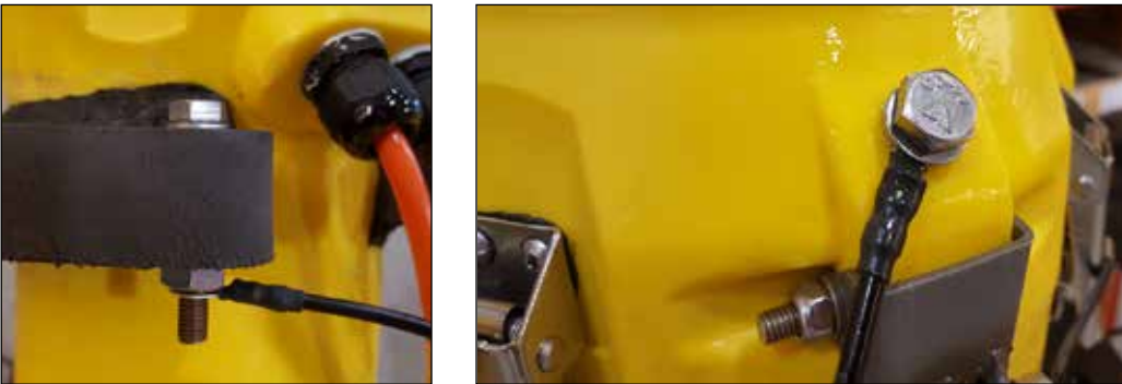
Illustration 12: Attaching the earthing cable
