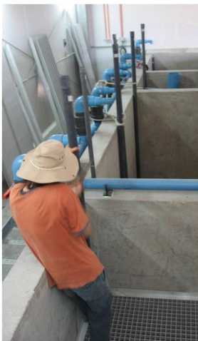
Installation of AKVA multi step bio filter, Chile
